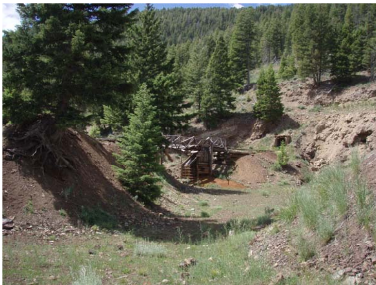
Photo #20 Three dangerously open adits remain on the Silver Dollar. There as apparently some redevelopment work that was conducted on these adits and a small ore bin/chute was constructed to ship some ore or samples (B. Schuld 7/22/10).
