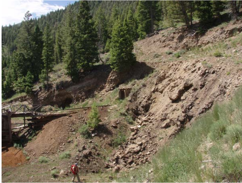
Photo #21 Three dangerous open adits remain on the Silver Dollar. There as apparently some redevelopment work that was conducted on these adits and a small ore bin/chute was constructed to ship some ore or bulk samples (B. Schuld 7/22/10).
