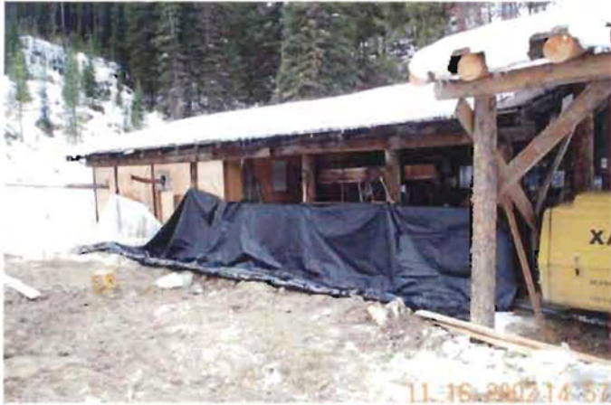
Photo 4: Pits filled in and pond liner placed against wall and over main concentration of spill. Sloped to drain toward front of building.
